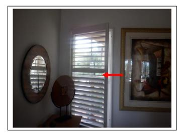
19. The master bedroom right window's top pane is fogged. This is an indication that the seal between the two panes of glass has failed. See the pictures below.
