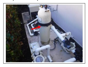
29. There is a hole in the pool heater case that is being patched by tape and screen. See the picture below.
