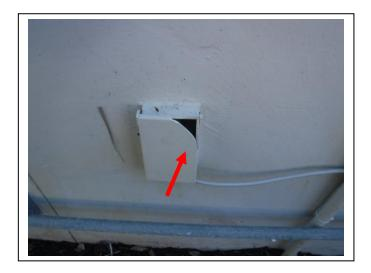
9. The exterior electrical outlet at the front right corner of the home is missing the weatherproof cover. See the picture below.
