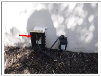
8. The exterior electrical outlet for the lawn sprinkler controller has a broken weatherproof cover. See the picture below.
